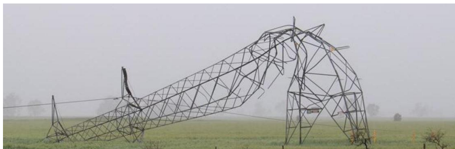
Wind failure of a power line support tower
